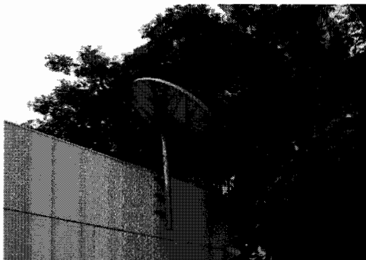
VSAT satellite dish to receive and transmit signals
